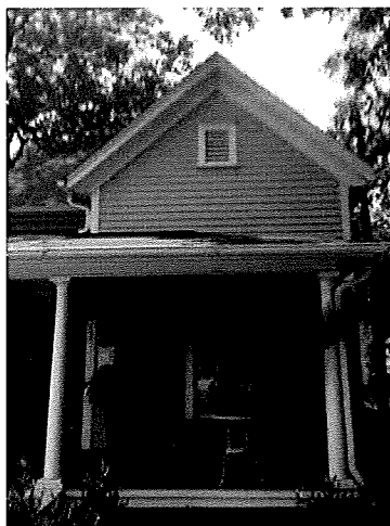
Vent in peak of sheds to match peak on front of house
