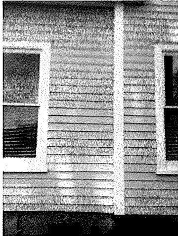
Sheathing will be wood siding. Trim to match main house.
